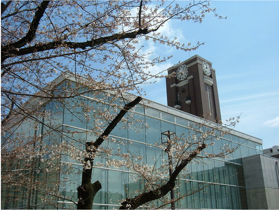
Kyoda's historical Clock Tower Centennial Hall
